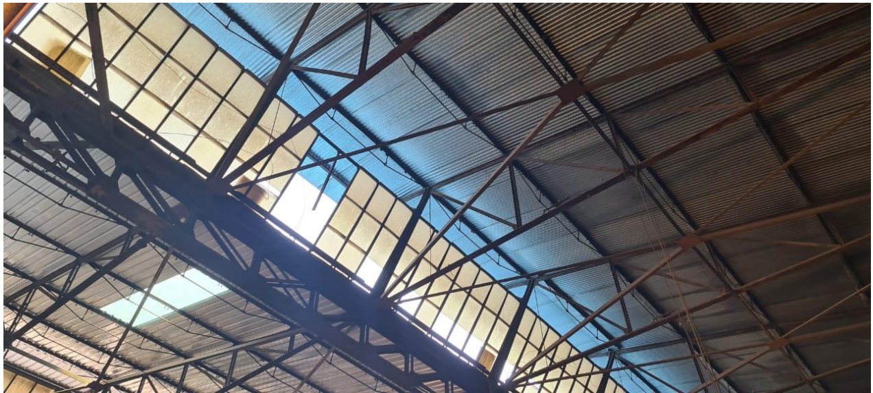
Replacement of Broken AC/GI Sheets in Shed A, B, Mill Wright, Machine Shop, Pit Line 1,2, 3 & C Ward in GSD Jhansi
