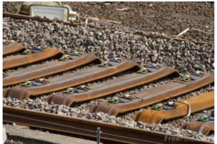
Steel Trough Sleepers
