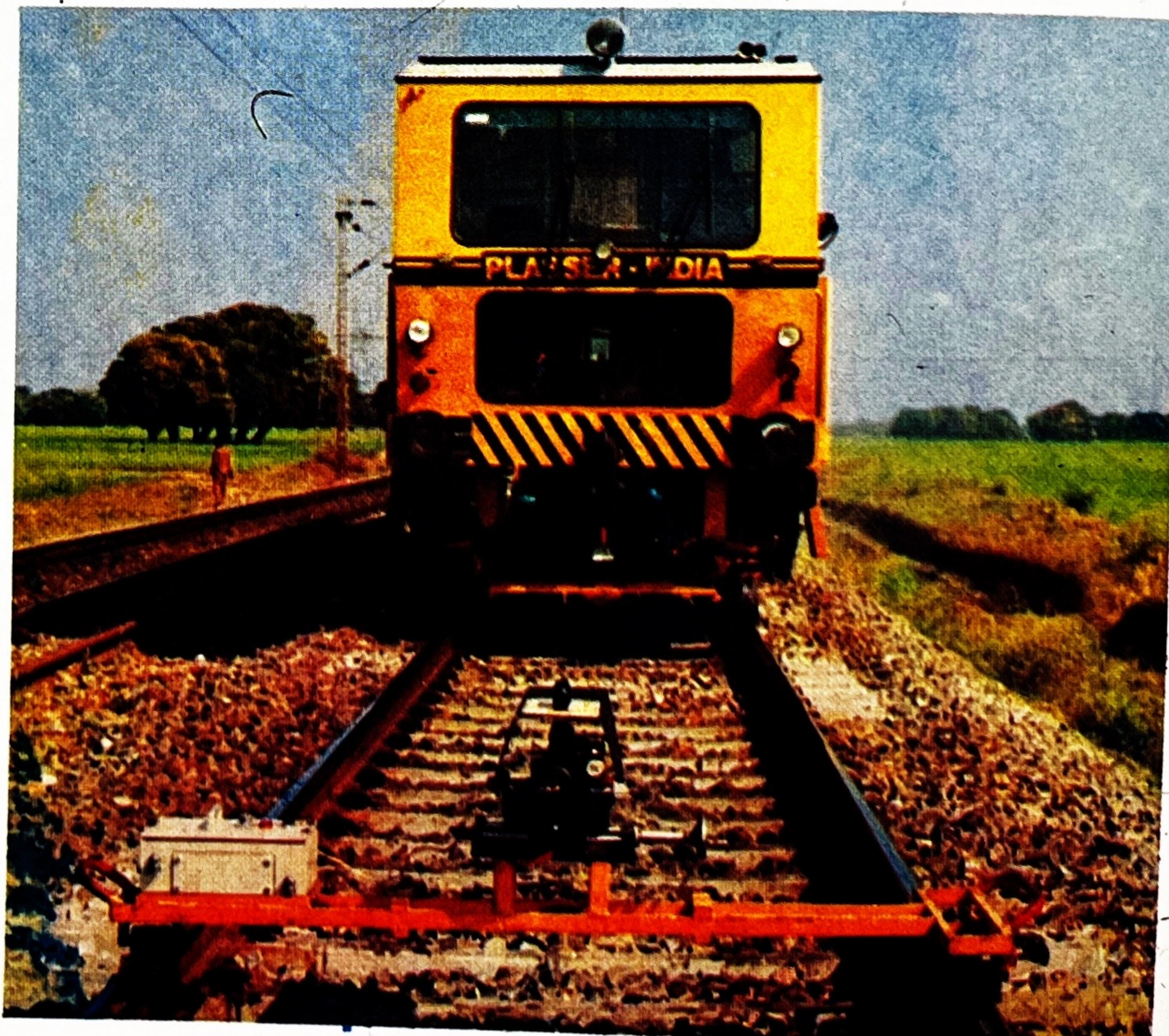
09 - 32CSM USING LASER BEAM FOR LINING
