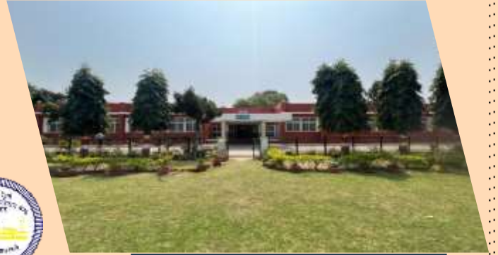
New Administrative Building
