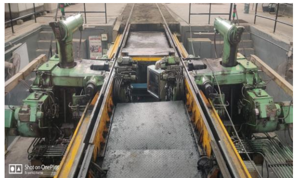
PIT WHEEL LATHE
