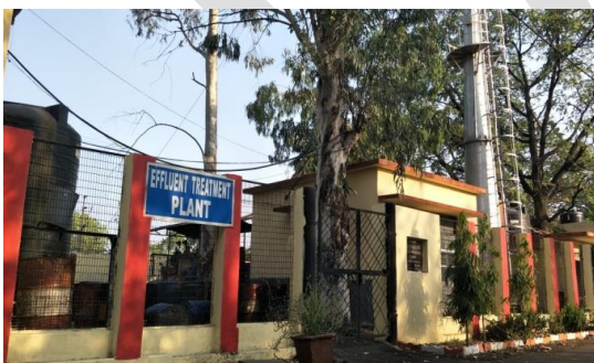
EFFLUENT TREATMENT PLANT
